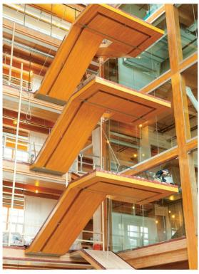
Safe and efficient connections and braces: Throughout the building, special connections were put in place to attach steel beams and wood beams to engineered wood columns. Diagonal glulam heavy timber braces at the end walls of each storey are used to resist seismic loads. Wood was a natural choice for the Earth Sciences
