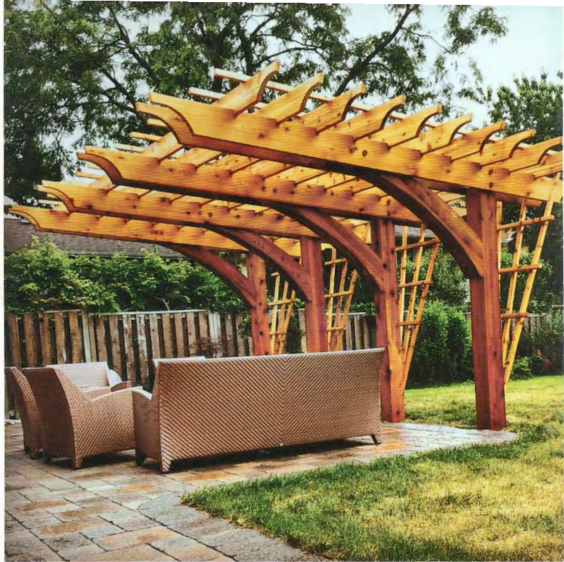
Any outdoor projects such as this pergola is ideal in Western Red Cedar – which is termite, rot and decay resistant
