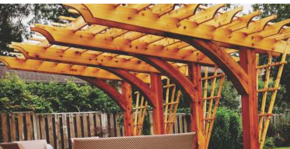
* Credit: Photo by churchvillecontracting.ca
