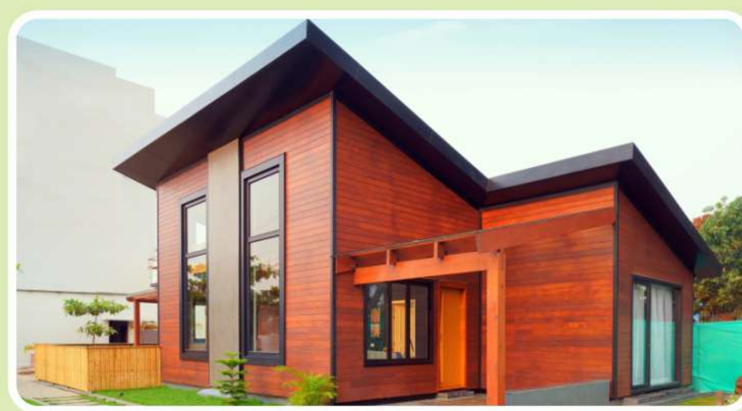
Single storey WFC house - Chennai, Tamil Nadu
