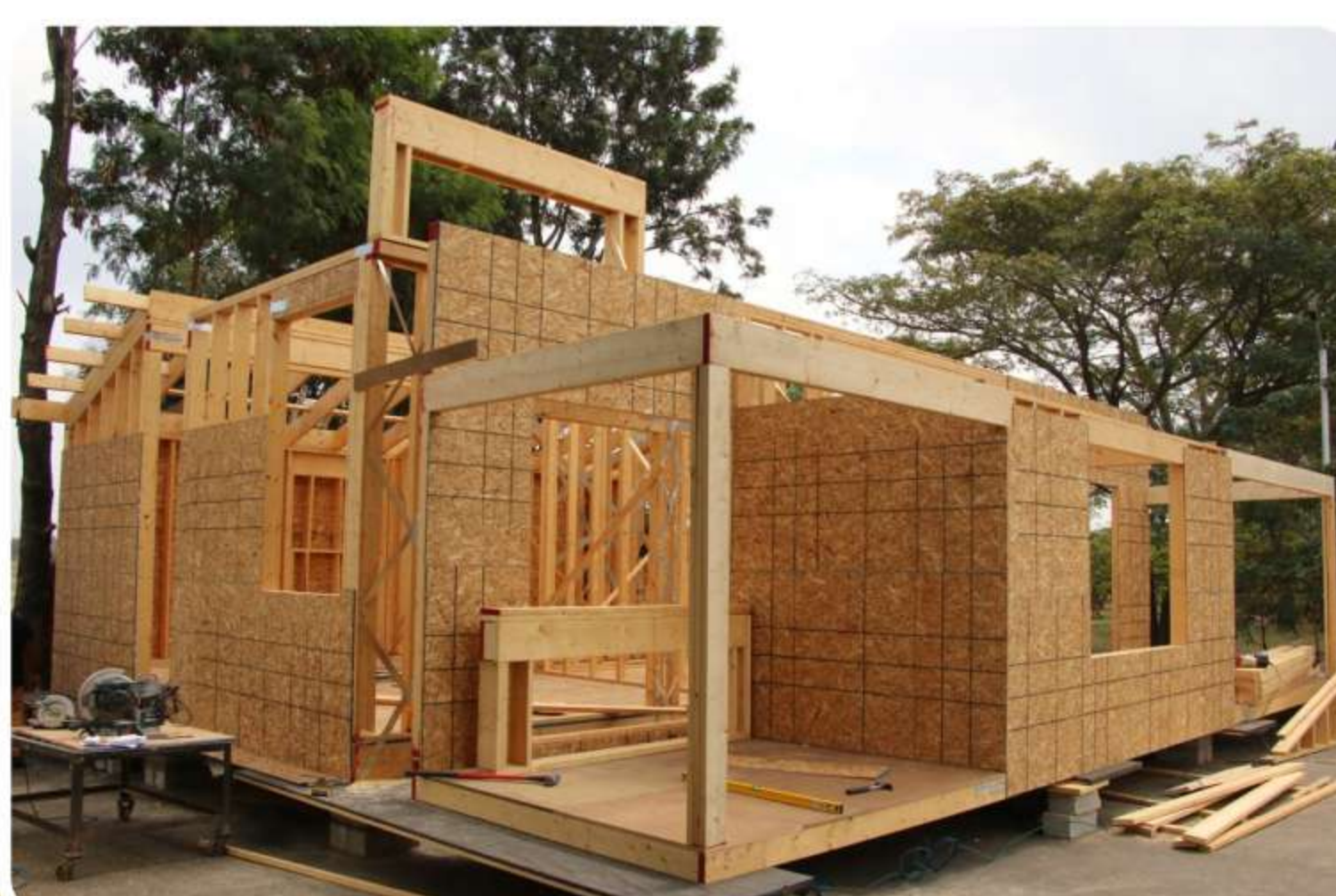
Wood Frame Construction in progress
