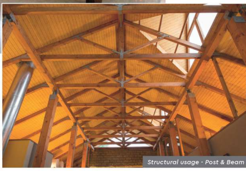
Structural usage - Post & Beam
