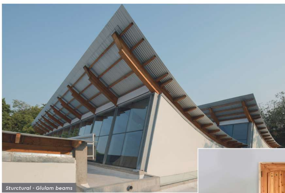
Structural - Glulam beams
