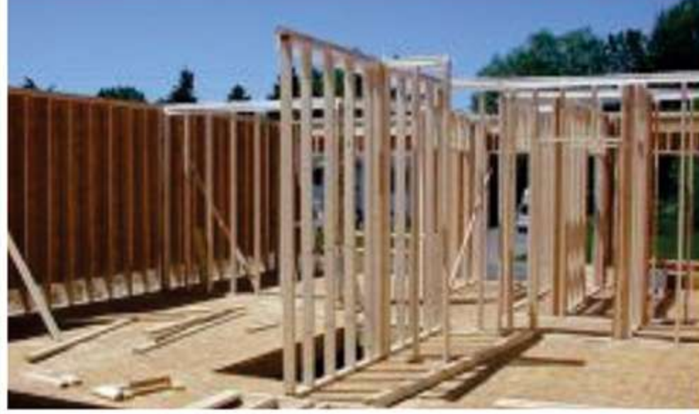
Wood Frame Construction in progress
