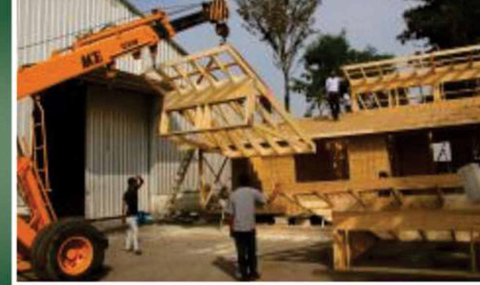
Wood Frame Construction in progress
