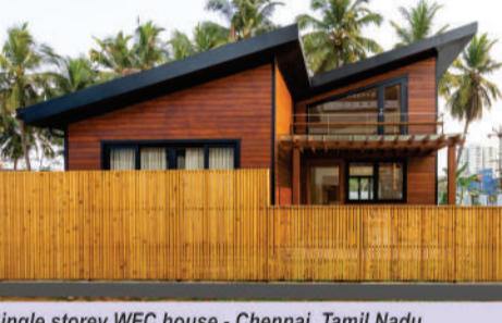
Single storey WFC house - Chennai, Tamil Nadu
