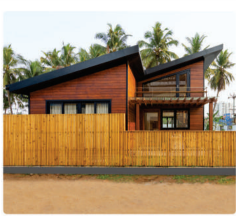
Single storey WFC house - Chennai, Tamil Nadu
